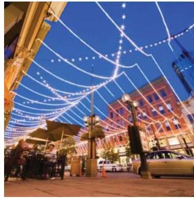
1.19 ENHANCED LIGHTING PILOT #1
